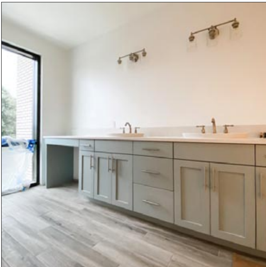
Main Bathroom Suite Progress — Photo: Studio Mas Creative
